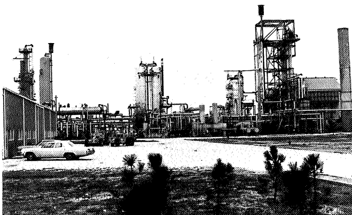
Figure 1. Typical 1,000 ton Kellogg ammonia plant using natural gas as feed.
